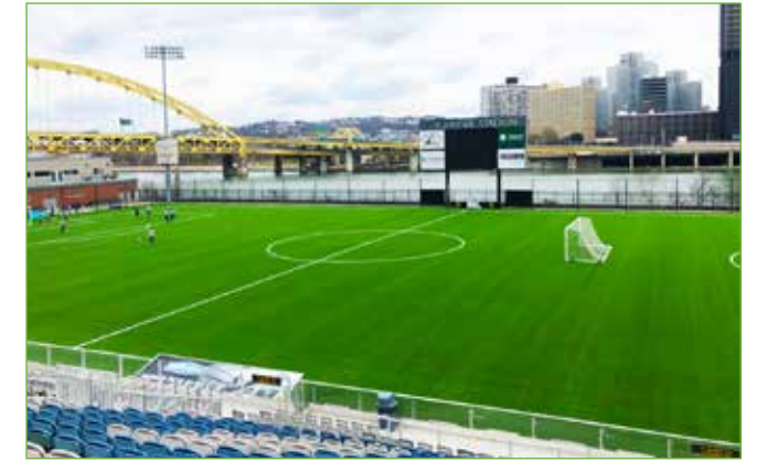
Highmark Stadium - Pittsburgh, PA
